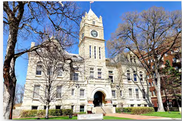
Figure 14 Riley County courthouse.
